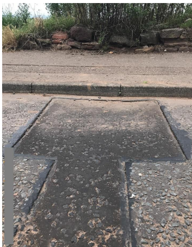
Picture 21 – Inadequate compaction of the unbound backfill?
