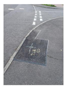
Marked Location Photographs show where the core is to be taken within the reinstatement. It is recommended that the framing of the photograph should be done in such a way that additional locational information can be accommodated at the same time.
