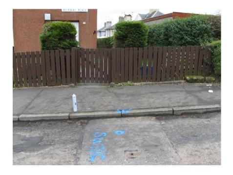
Marked Location Photographs show where the core is to be taken within the reinstatement. It is recommended that the framing of the photograph should be done in such a way that additional locational information can be accommodated at the same time.
